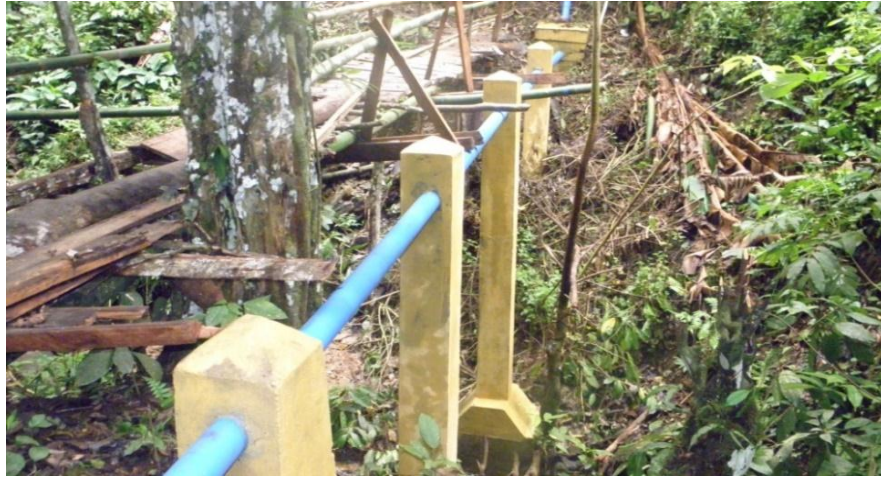
Gambar III.33. Jaringan Pipa Transmisi
