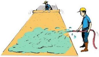
Gambar 3.30 Curing Beton
