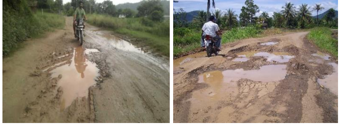
Gambar III.28 Lubang ( Pot Holes )
