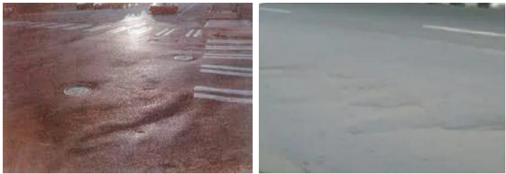
Gambar III.22 Keriting (Corrugations)
