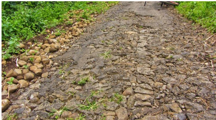
Gambar III.30 Aus (Wearing)
