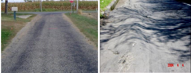
Gambar III.16 Kegemukan Aspal ( Bleeding )
