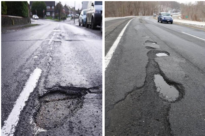
Gambar III.23 Lubang lubang ( Pot Holes )
