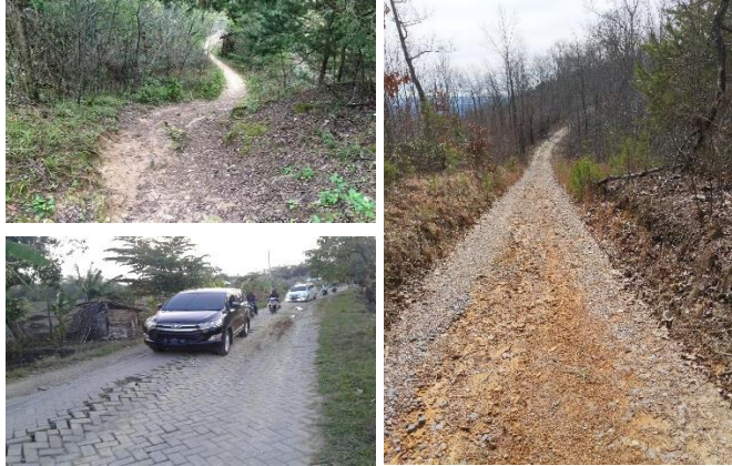
Gambar III.26 Alur ( Rutting )
