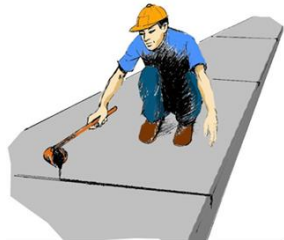
Gambar 3.24 Pengisian Joint Sealent
