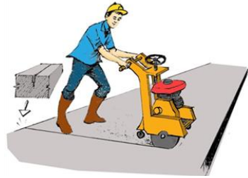
Gambar 3.23 Cuting Beton
